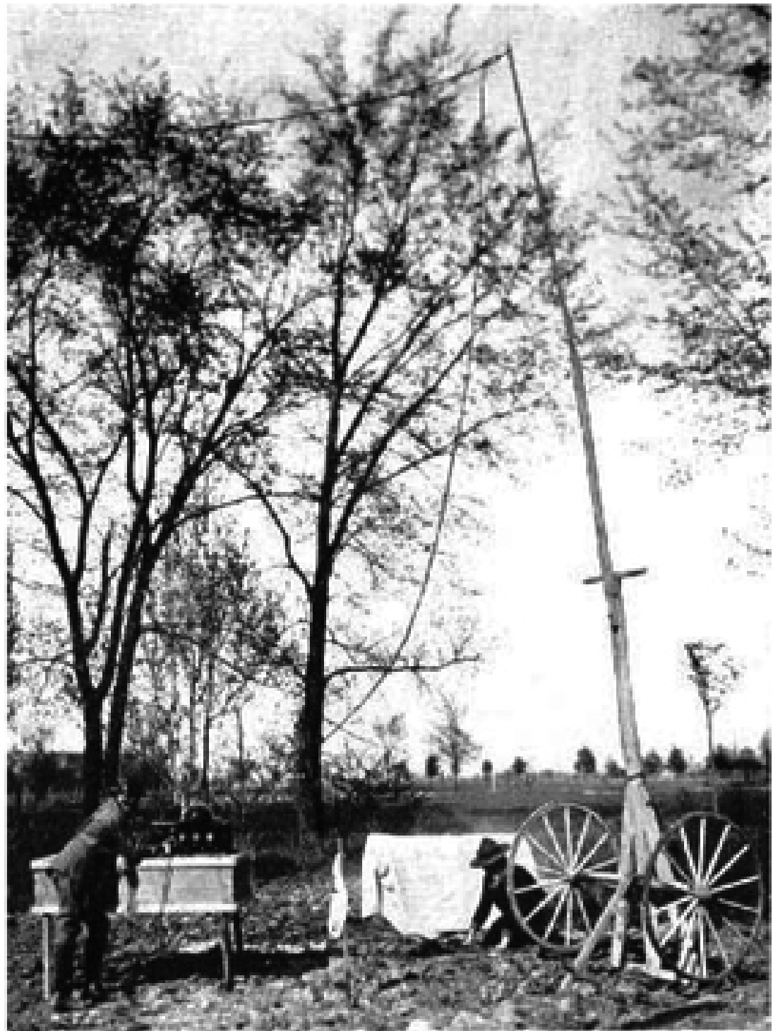
Knocked Down, The Trek Cart, Forms a Table, a Shelter, and an Aerial Radio Mast. - 1908
